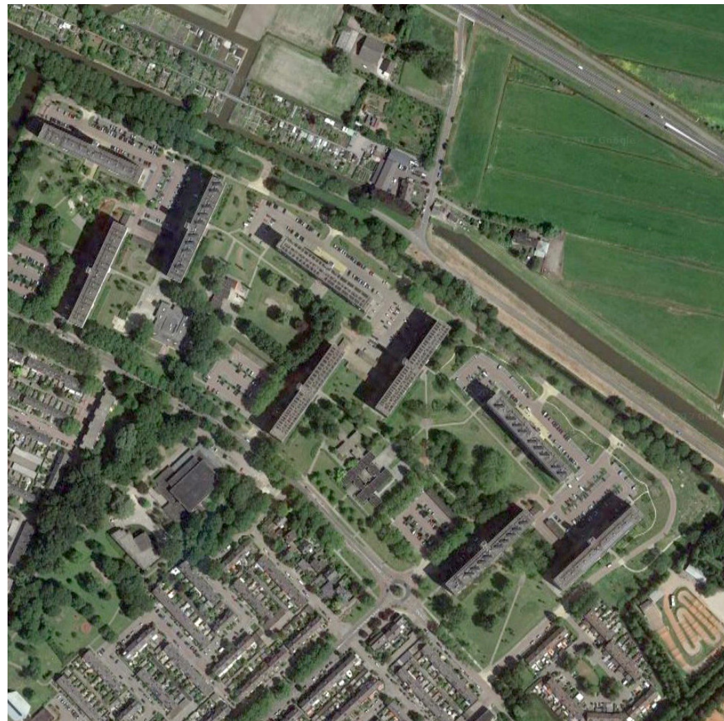
Aerial view 2017 © 2017 Google Maps
