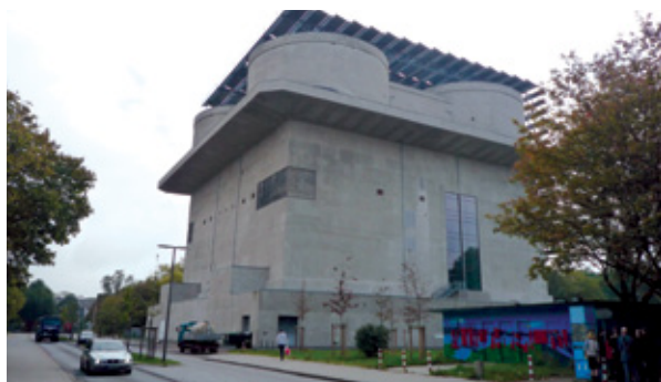
Figure 2. IBA Hamburg, Wilhelmsburg: Energy Bunker
