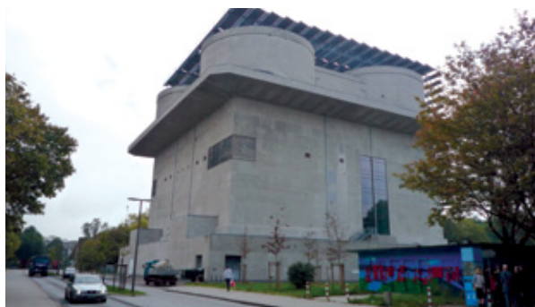
Figure 2. IBA Hamburg, Wilhelmsburg: Energy Bunker
