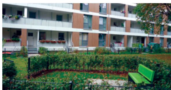
Figure 3. IBA Hamburg, Wilhelmsburg: retrofitted mix-tenure housing and common green areas
